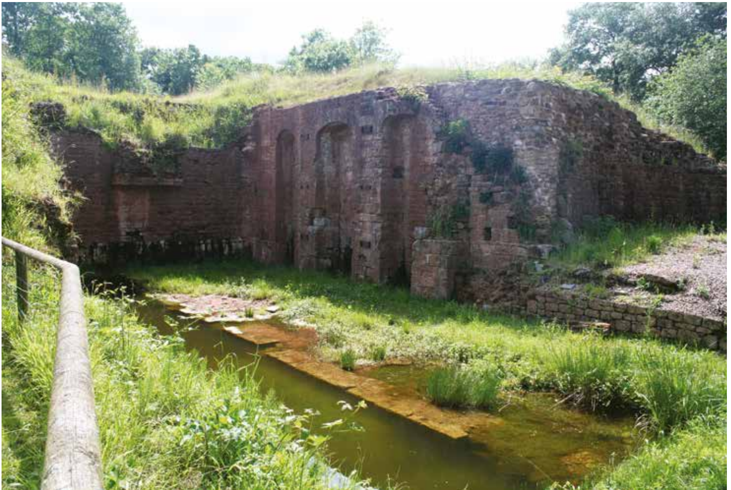
The remains of the Nynehead Boat Lift. The stone walls were part of the caisson chambers while to the fore were the locks at the entrance to the chambers.
