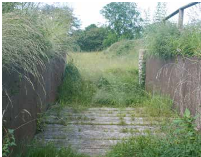
Access to the top chamber of the lift is via the old channel over the aqueduct. Note the iron sides to the channel.
