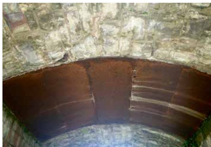
The iron plate in the middle of the aqueduct arch.
