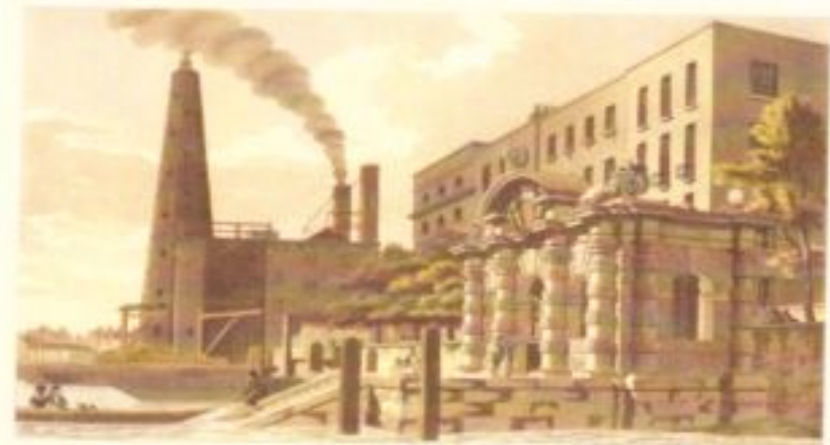
The Watergate, the York Buildings Company centre of operations on the Thames.
