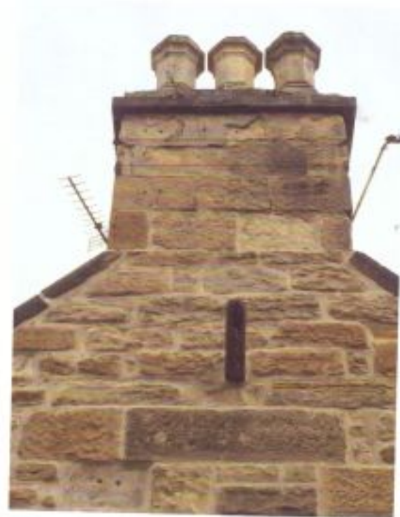
Stone sleeper blocks built into the wall of a local house, circa 1862.
