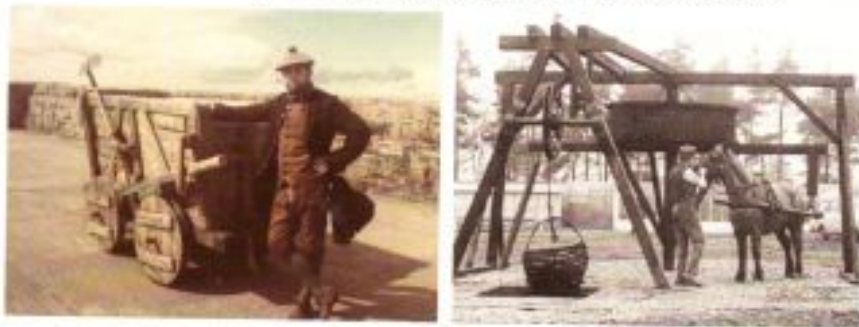
Wooden waggons & coal gin mechanisms were used on the early waggonway
