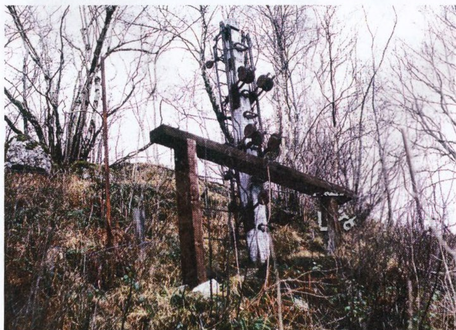
The Pass of Brander stone signals (also known as Anderson's Piano due to their use of tensioned wires) were first brought into use in 1882, to warn of rockfalls on this section of the Oban branch of the West Highland Line. GAVIN MORRISON.
