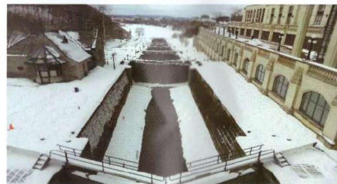
RIDEAU CANAL, OTTAWA, CANADA completed in 1832 a distance of 202 km with forty-seven locks.
