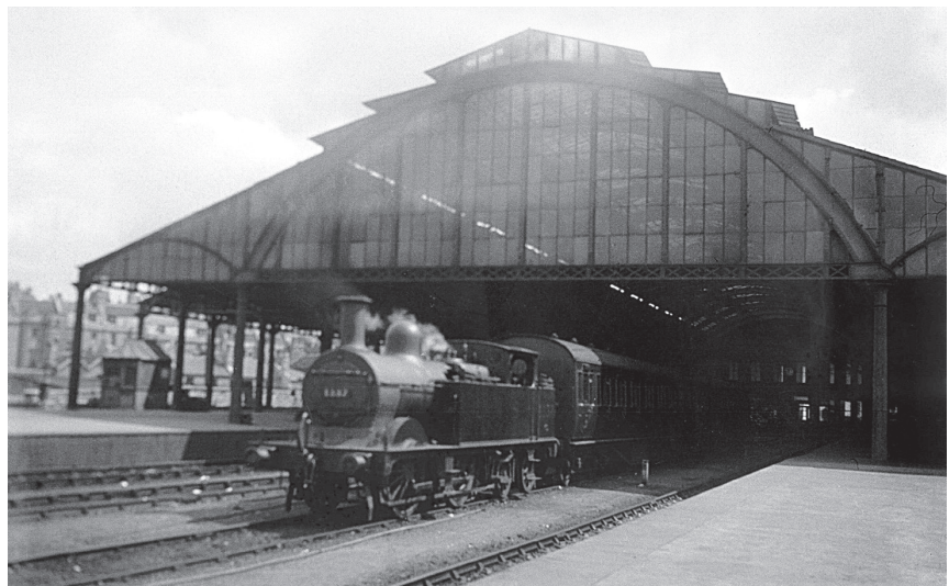
A late-1920s scene shows the glazed end of the train shed to good effect. As at St Pancras (opened the year prior to Bath), the supporting pillars to the main central span were grounded onto basement piers, the spacing of which enabled barrels of Bass beer (and other bonded goods) to be stored in bays under the north platform. IVO PETERS, COURTESY JULIAN PETERS
