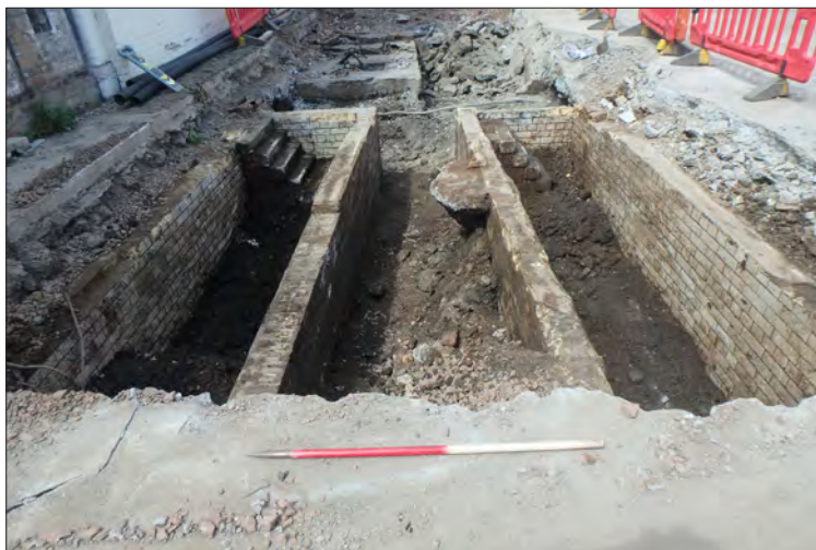
Plate 41: Brick-built maintenance chambers (8904) for Trams
