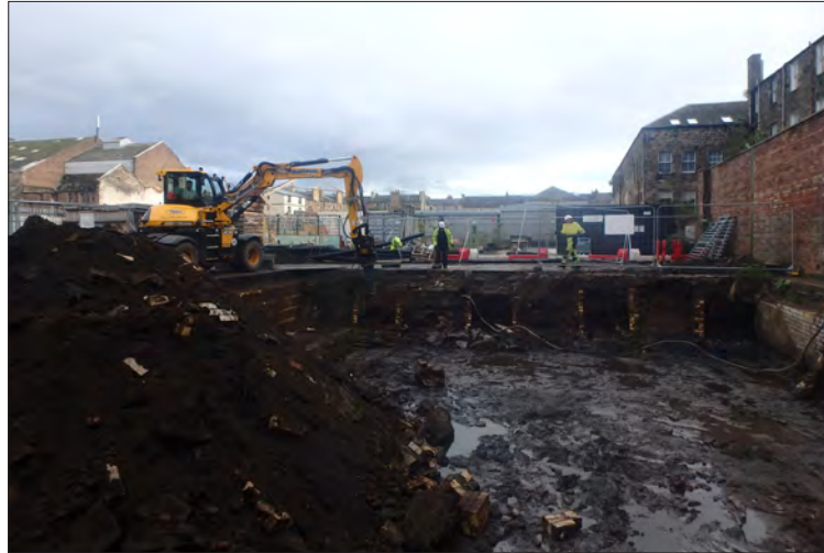
Plate 42: General view of excavation trench for new sub-station after chambers removed
