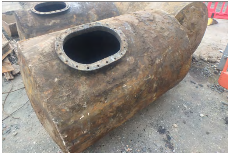
Plate 43: Old fuel tanks recovered during the excavation for the new sub-station
