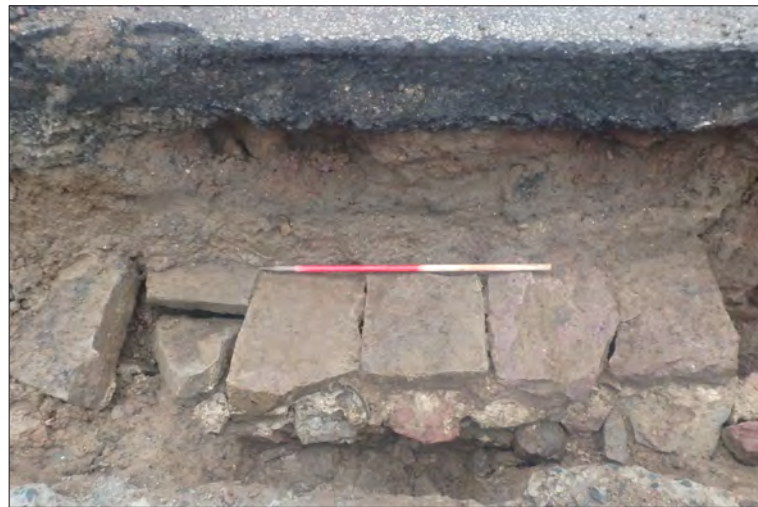
Plate 48: Flat capstone culvert (0315) at Antigua St
