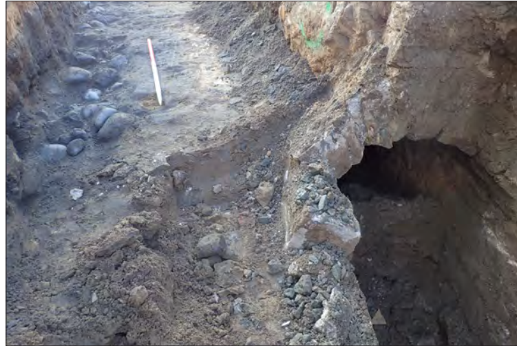
Plate 11: Detail of relationship between open drain and later main culvert
