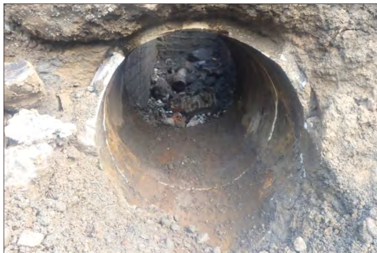
Plate 25: Detail of cable tunnel built from glazed tiles.
