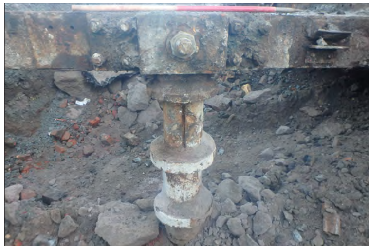
Plate 27: Horizontal beam and pillar associated to the cables tunnel at Antigua Street/Baxter's Place
