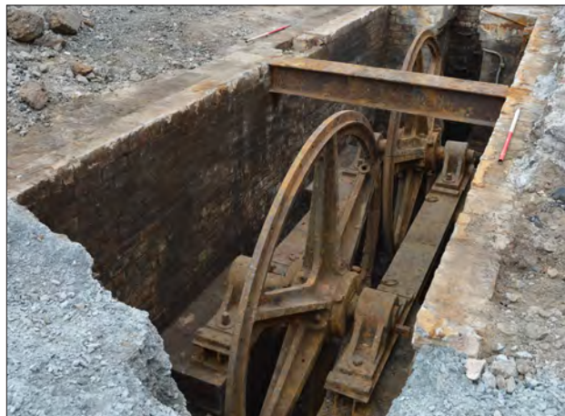
Plate 36: General view of the wheel house (7016)
