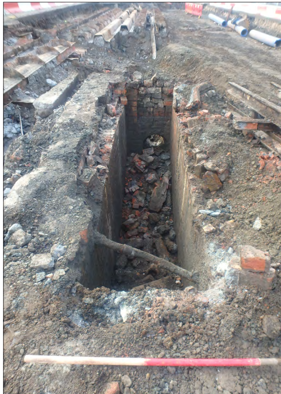
Plate 24: Cable tunnel running north-east/south-west.
