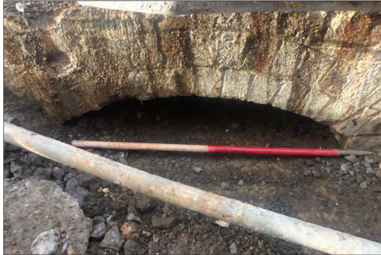
Plate 23: Entrance to the small corridor that communicate the parallel cable tunnels
