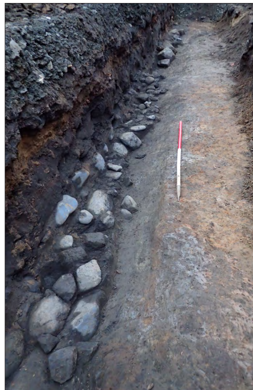
Plate 10: Section 62, open drain (6051) along edge of the road in the duct bank trench
