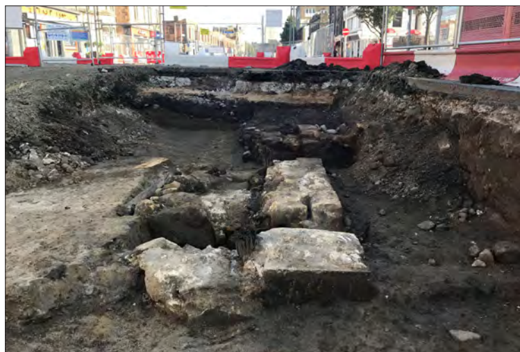
Plate 5: Stone foundation (6012) with drain and section, from the south
