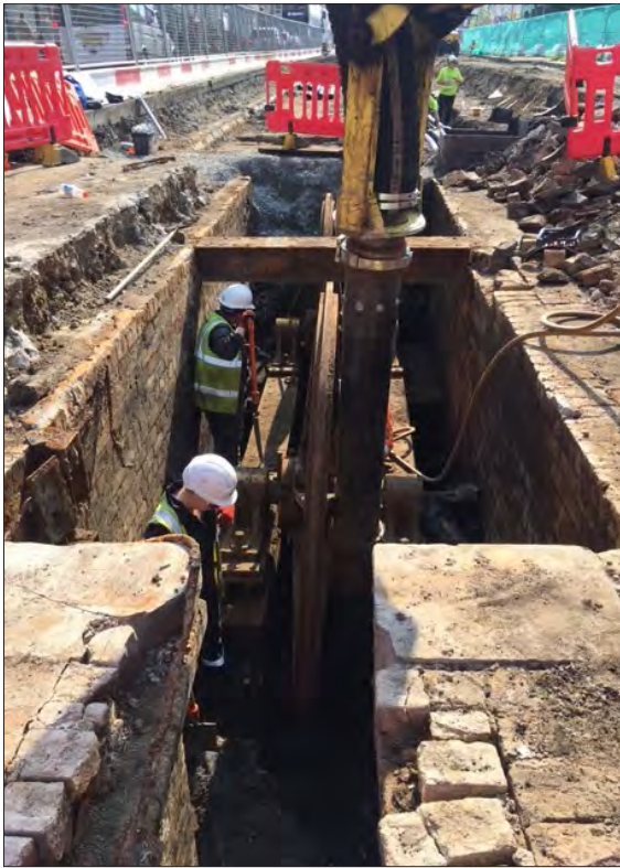
Plate 37: Completing the excavation of the Wheelhouse, from the North
