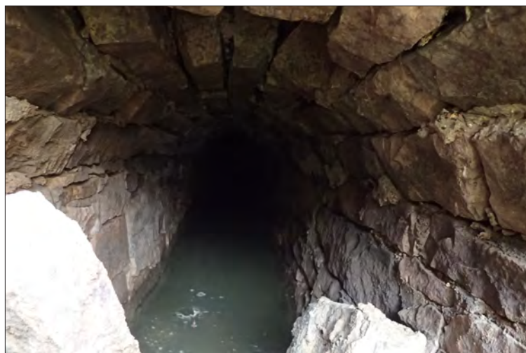
Plate 51: Inside view of the main arched culvert in Section 75
