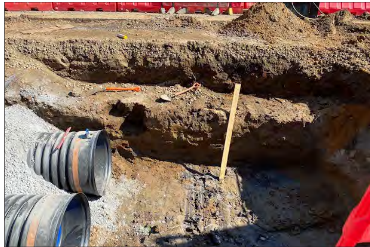
Plate 52: Construction of the attenuation tank on Iona Street
