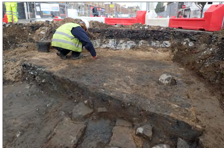
Plate 15: Cleaning, top surface of the road at Area 60
