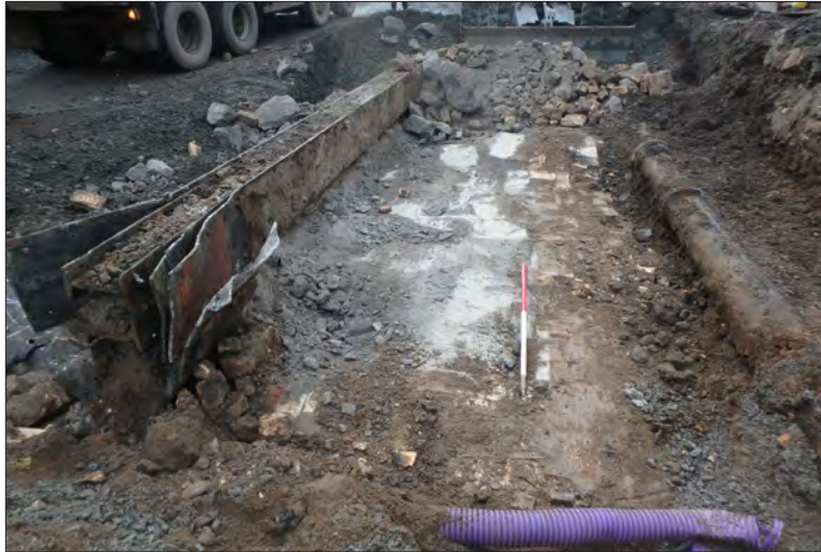
Plate 33: Horizontal central beam uncovered inside the cable housing
