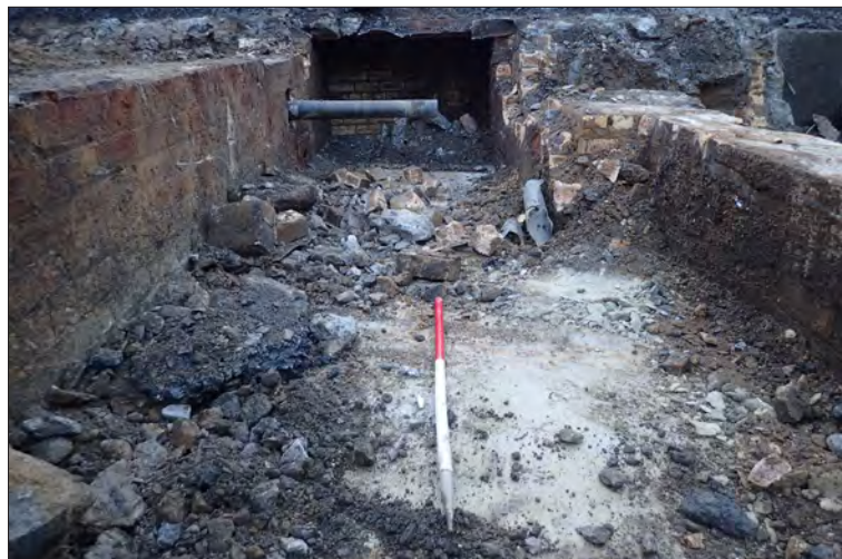
Plate 31: Area 73, inside detail of cable tunnel (7314)
