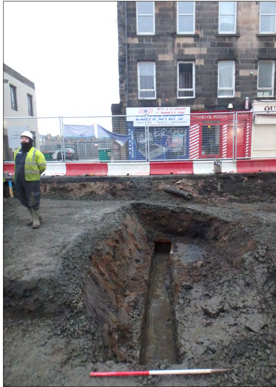
Plate 49: Location culvert (6226) with a square section and no surviving capstones
