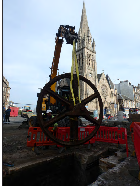
Plate 38: Wheels being removed in advance of conservation treatment
