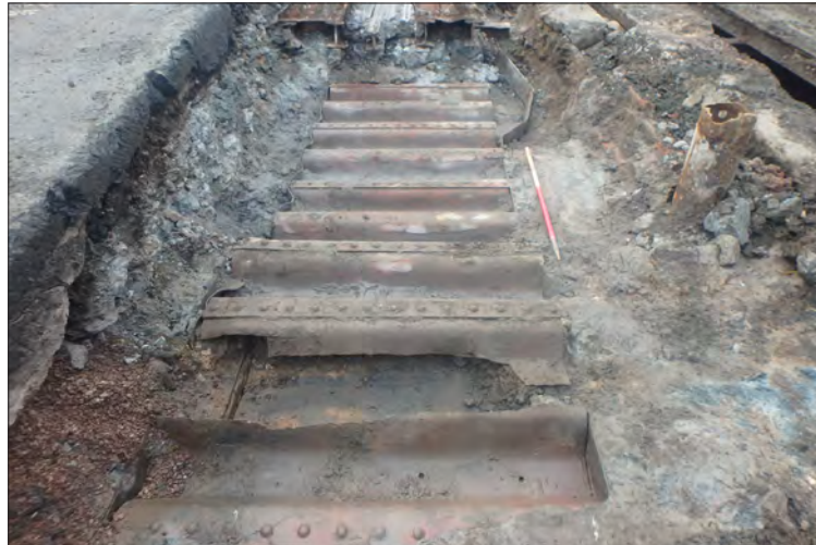
Plate 26: Plan view of cables tunnel (0323) taken from north-east
