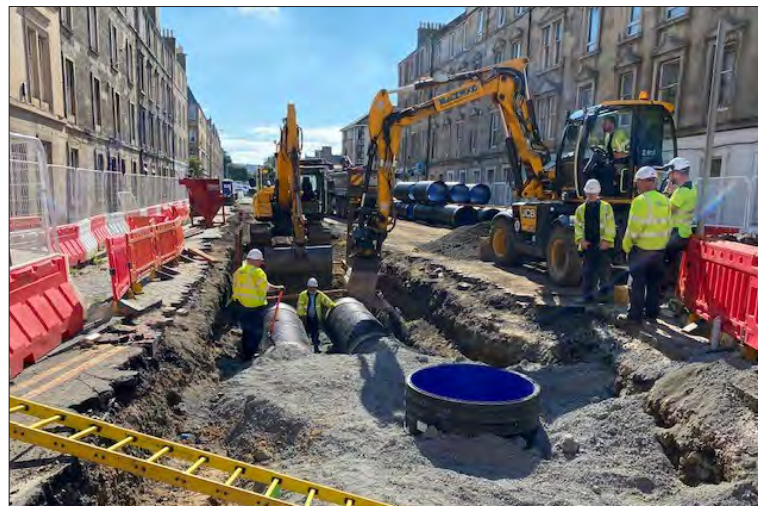
Plate 53: Attenuation tank on Iona Street, detail of natural sand deposits
