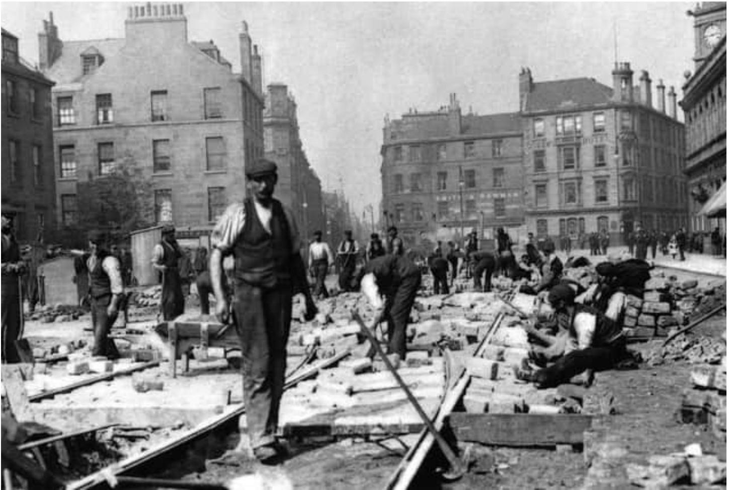
Long before the Trams to Newhaven project, construction workers installed the original tram lines on Leith Walk in 1904.
