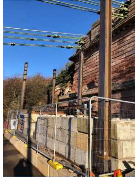
English access tower foundations (Spencer)
