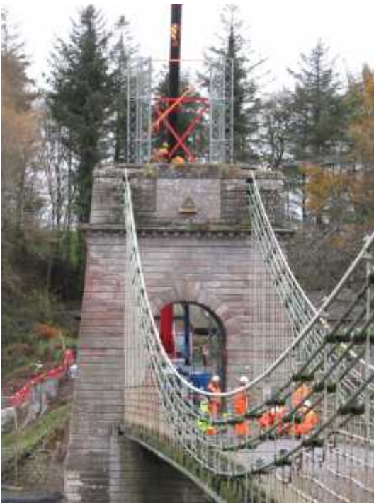
Erection of Scottish cableway tower and removal of decking (foreground) Friends
