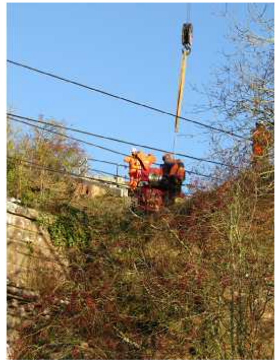
Installation of Woodliner cable crane above the English tower Friends
