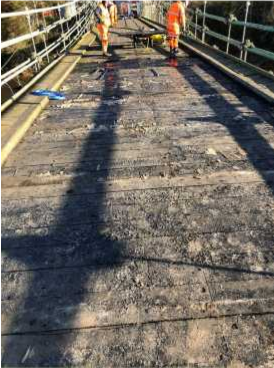
Removal of decking plywood (Spencer)
