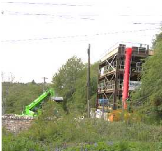
The English tower behind structural steel access platform - 19 th May 2021
