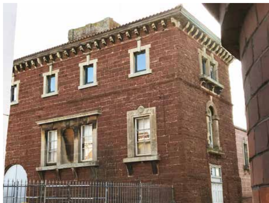
Seen from the road is the former engine house, still an ornate building. The boiler house is just visible to the right.
