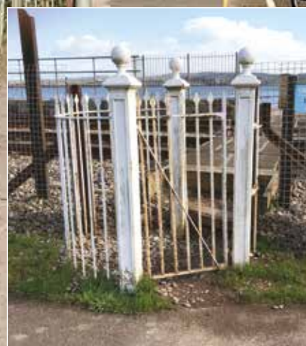
One of the foot crossings over the railway with cast iron posts and bridge rail supports for the fencing.
