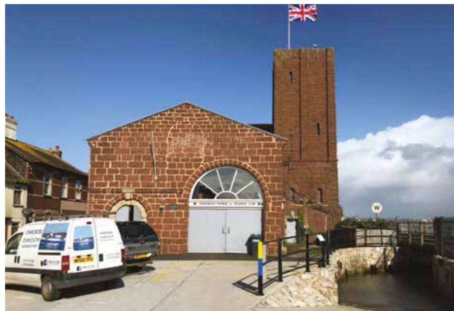
Today the pumping engine house is home to the local fishing and cruising club. This is the old boiler house.
